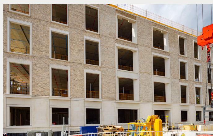
Progression of the facade installation on Building 5. Top: Facade above the hoarding line on Ordnance Hill. Bottom: Southern facade from within the site.
